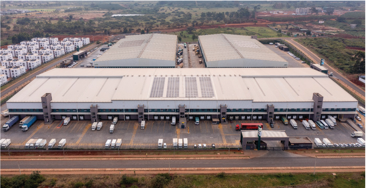
Figure 43: Photo of ALP North Three
